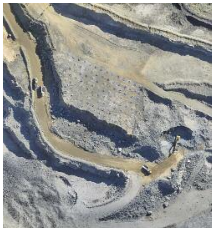
BME blast analysis: an aerial view from a camera mounted on a UAV clearly showing the blasting pattern
